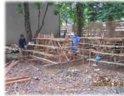
Local community enterprise—building plant risers.
